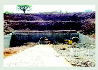
Construction of an underground mine and plant with a capacity of 3000 tpd near Pulivendula in Kadapa district of Andhra Pradesh is progressing satisfactorily. The mine entry is being constructed with three declines with ore planned to be hoisted through a conveyor. The plant shall have alkali leaching process under pressure. The project is expected to be commissioned during the year 2011.
